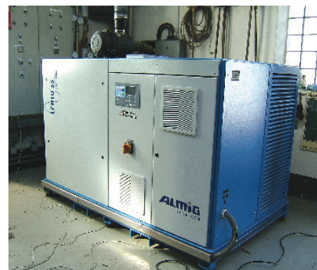
The LENTO 55 water-injected compressor, offering a volume flow of 7.9 m 3 /min has been up and running in the brewery since the summer of 2010
