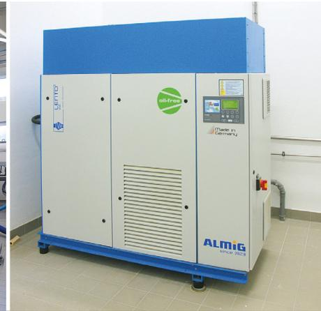
**03** Prolupin, based in Grimmen, northern Germany, generates the compressed air needed for various stages of production with a compressing Lento screw compressor which is absolutely oil-free right from the outset
